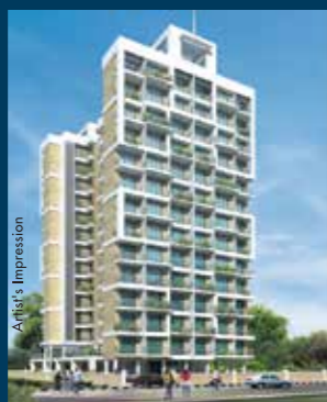
SAI GANGA ULWE G+13 Storeyed Tower
