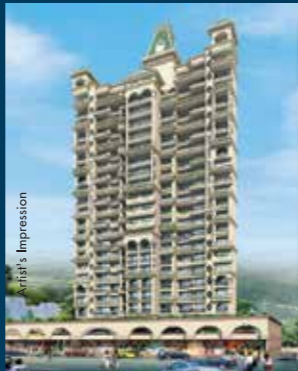
SAI MOKSH KHARGHAR G+22 Storeyed Tower
