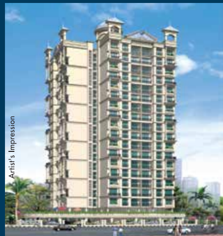
SAI JEWEL KHARGHAR G+18 Storeyed Tower
