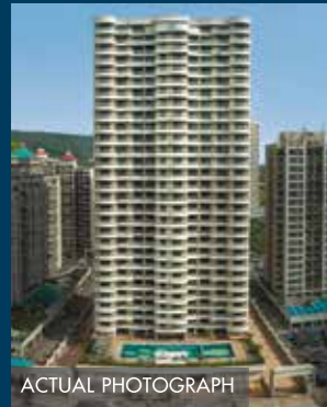
SAI SPRING KHARGHAR G+29 Storeyed Tower
