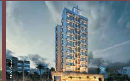
SAI AARADHYA KHARGHAR G+21 Storeyed Tower
