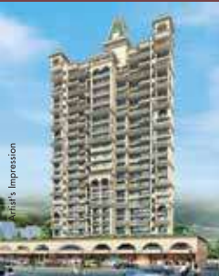
SAI MOKSH KHARGHAR G+22 Storeyed Tower
