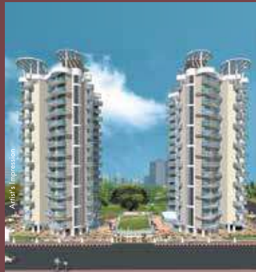
SAI PEARLS KHARGHAR G+15 Storeyed 2 Towers
