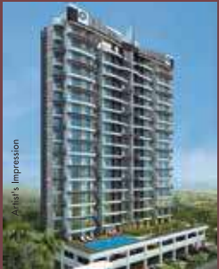
SAI WONDER KHARGHAR G+18 Storeyed Tower
